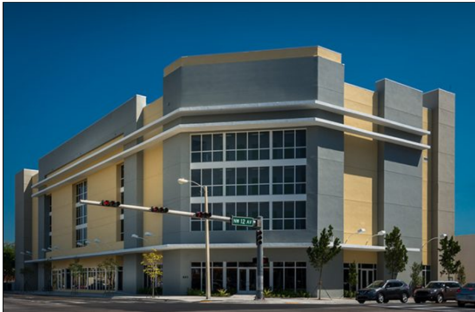
641 Northwest 12th Avenue
